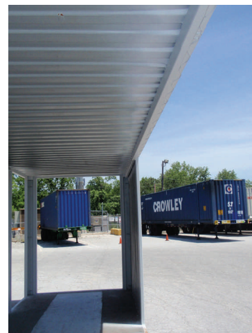
One of the fabricated sections for the shipping container house being by a design + construction, llc 404-992-8605
